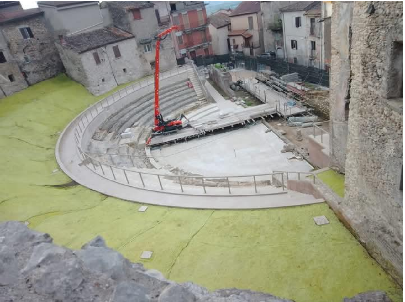
Ferentino, 12th May 2025, Roman theatre restoration work
